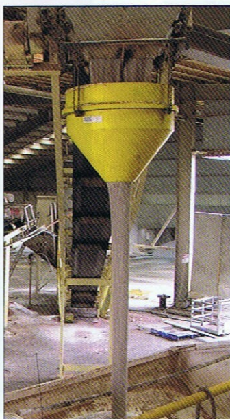
The Dust Suppression Hopper in action.
