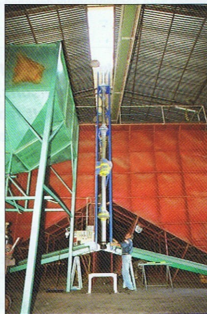
Installation of an Olds Elevator.
